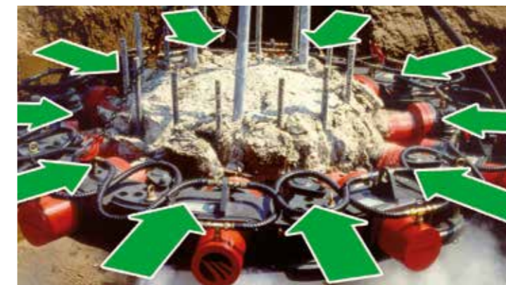
Activating the oilflow, PB crushes the concrete part without damaging the lower structure
