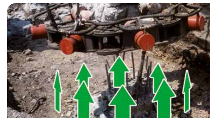
Lifting up, PB takes out the concrete and leaves the steel rods free
