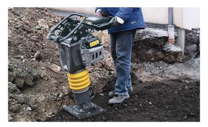
\*BOMAG tampers with Honda GXR 120 petrol engines (**BT 60** and **BT 65**) can also be used in trenches deeper than shoulder height and at least 1.5 m wide. Further information at: www.bgbau.de (BG Bau, Deutschland, 2015).
